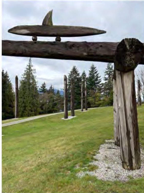
Unit #2, "The Direction", is noted as in need of monitoring on a regular basis.
