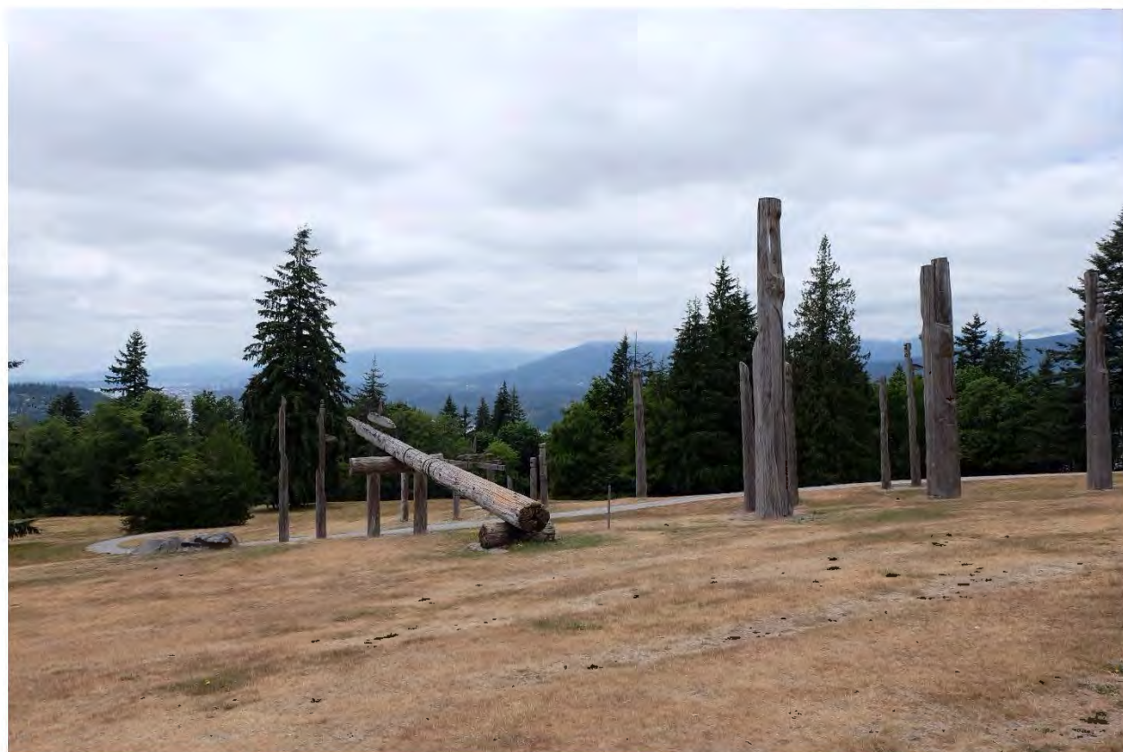
Overall, of the western slope of the site, Unit #2, “The Direction”, centre, is noted as in need of monitoring on a regular basis.
