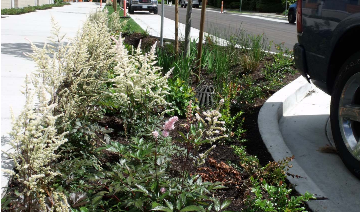
Figure 7: Curb Bulge with Rain Garden
