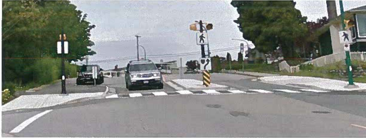
Figure 5: Existing Roadside-mounted Special Crosswalk at Beta Ave/Brentwood Dr
