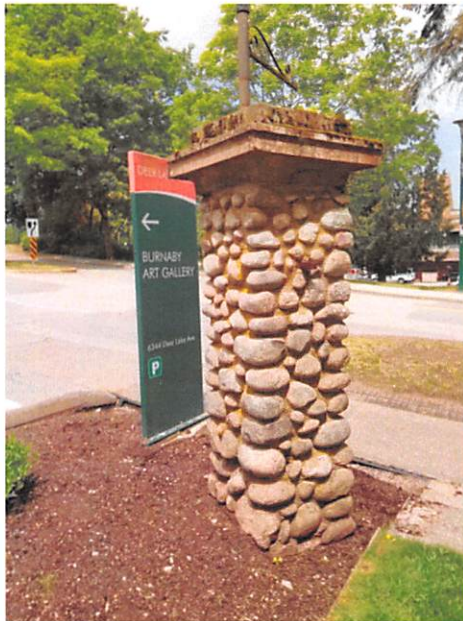
Cobblestone gate pillar. Note the anchor metal anchor that would have supported a metal gate.
