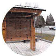
Example use of wood infrastructure on site at Burn Lake Park
