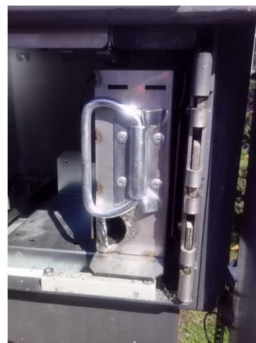
Damaged parking meter
