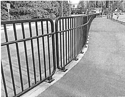
Photograph #5: Typical 1.4m high bicycle fence at the curb with a 1.2m high handlebar rub and hand rail.
