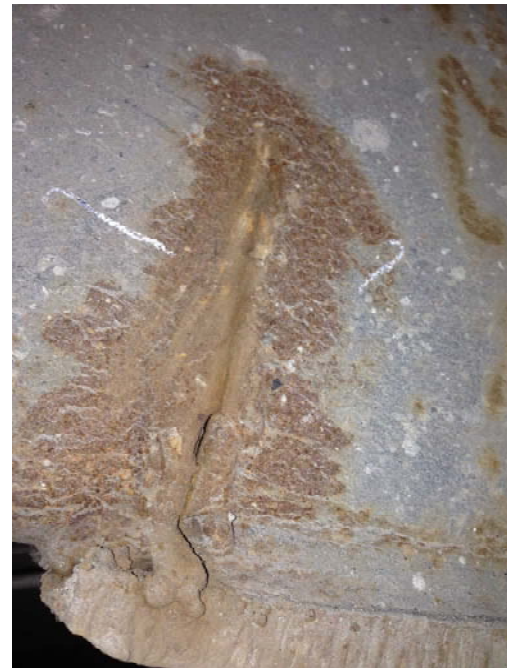
Cracked frame found on dump truck taken out of service, Feb. 25.
