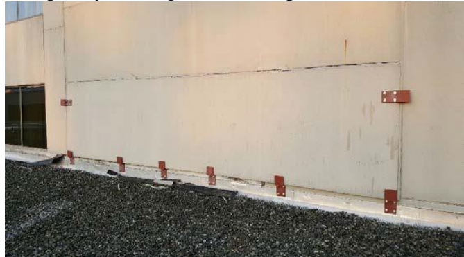
Temporary bracing – interim repair:
