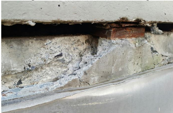
Close-up view of deteriorated curbing:
