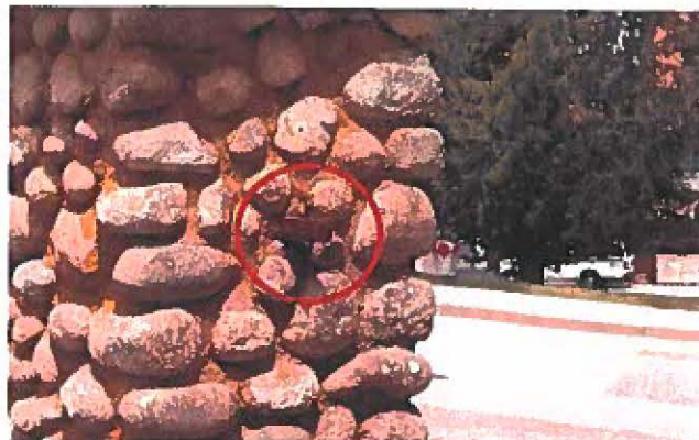
Cobblestone gate pillar. Note the anchor metal anchor that would have supported a metal gate.
