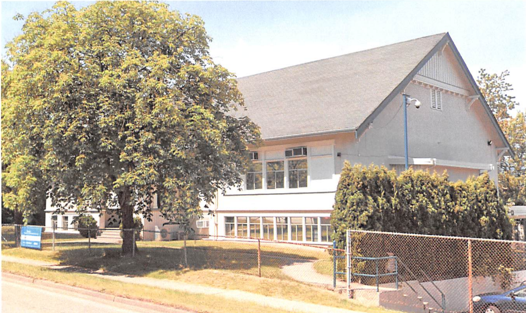
Pre-restoration condition of the school. The conservation project will re-instate the original design of the building's windows. The gable end features intact wood work detailing which will be retained and restored.
