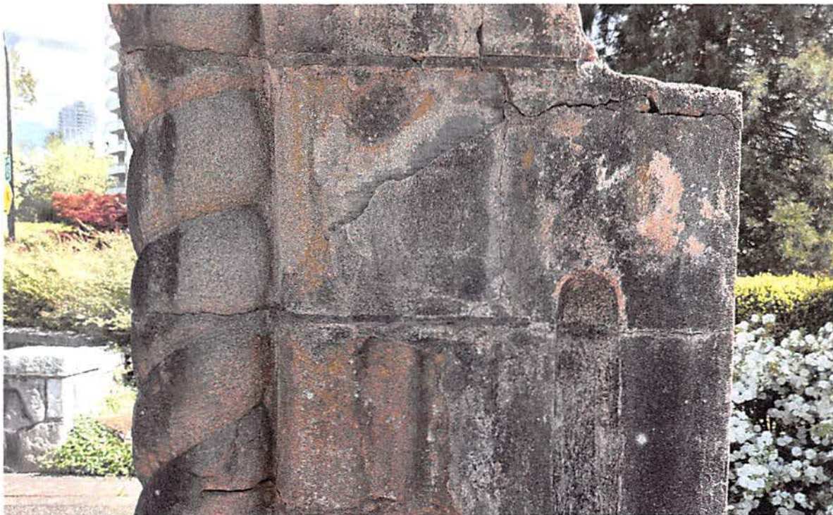
Detail image of area to be repaired through repointing of masonry and stabilization to prevent fractures
