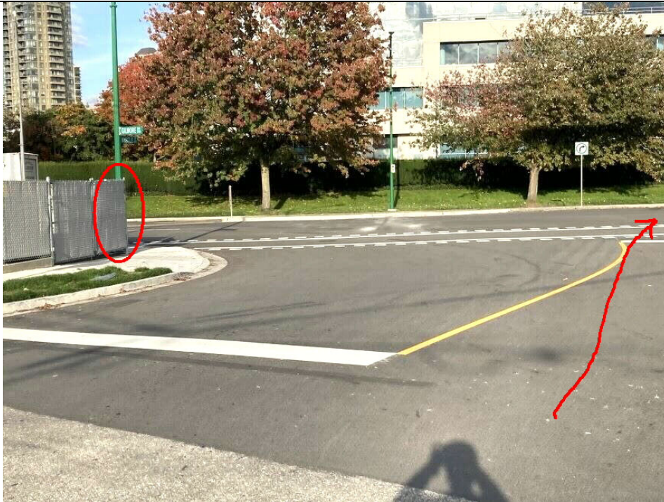
Intersection of Myrtle and Gilmore. Drivers heading east on Myrtle to turn right onto Gilmore have their sightlines to southbound cyclists obscured by tall fencing (opaque due to privacy slats)
