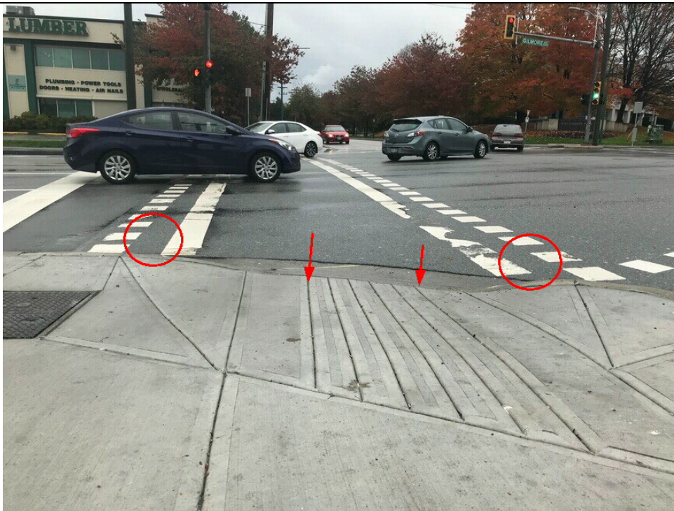
Crosswalk over Gilmore Ave at north end of Still Creek Ave. Arrows at elephant's feet indicate width of curb cut. Circles indicate width of a safe comfortable curb cut for cyclists.
