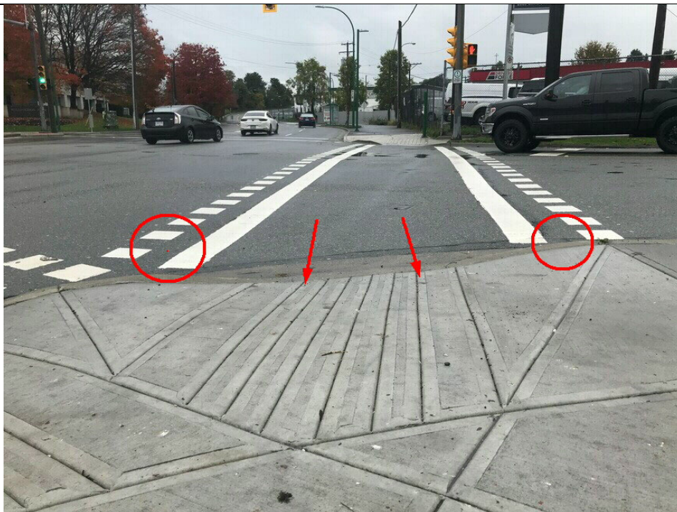
Crosswalk over Still Creek on west side of Gilmore. Arrows at elephant's feet indicate width of curb cut. Circles indicate width of a safe comfortable curb cut for cyclists.
