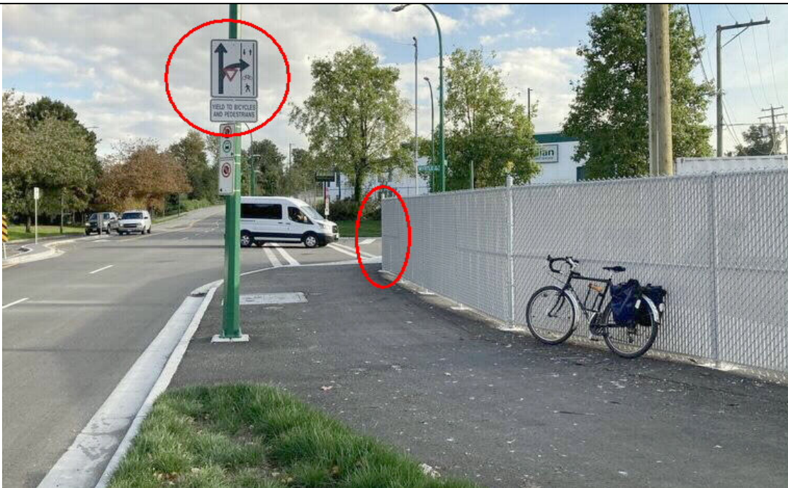
Southbound cyclists approaching Myrtle have their view of eastbound drivers obscured by fencing. The crosswalk has “elephant’s feet” markings so a southbound cyclist (conventional or E-bike) could enter the intersection at some speed and appear “out of
