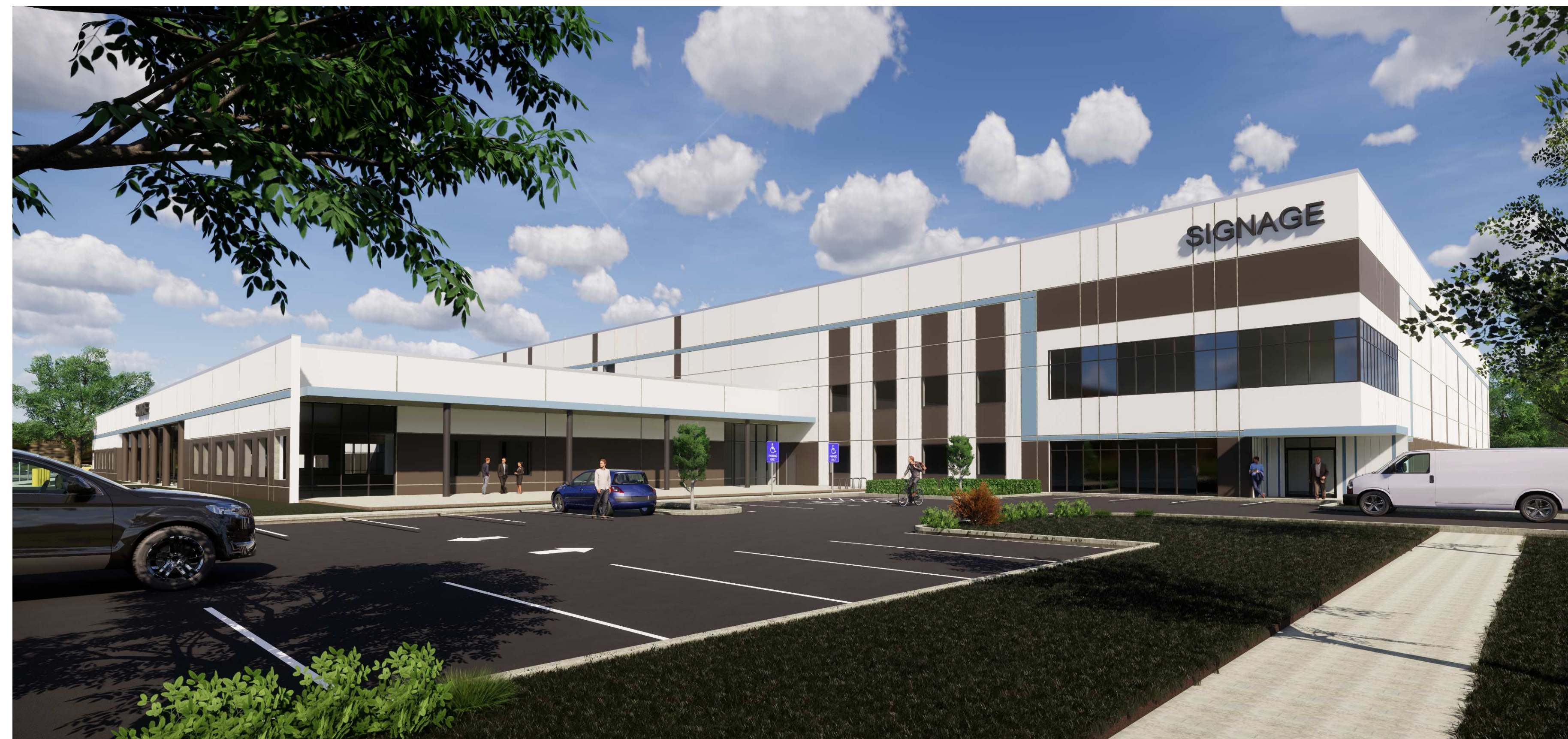
SOUTH-WEST CORNER VIEW
