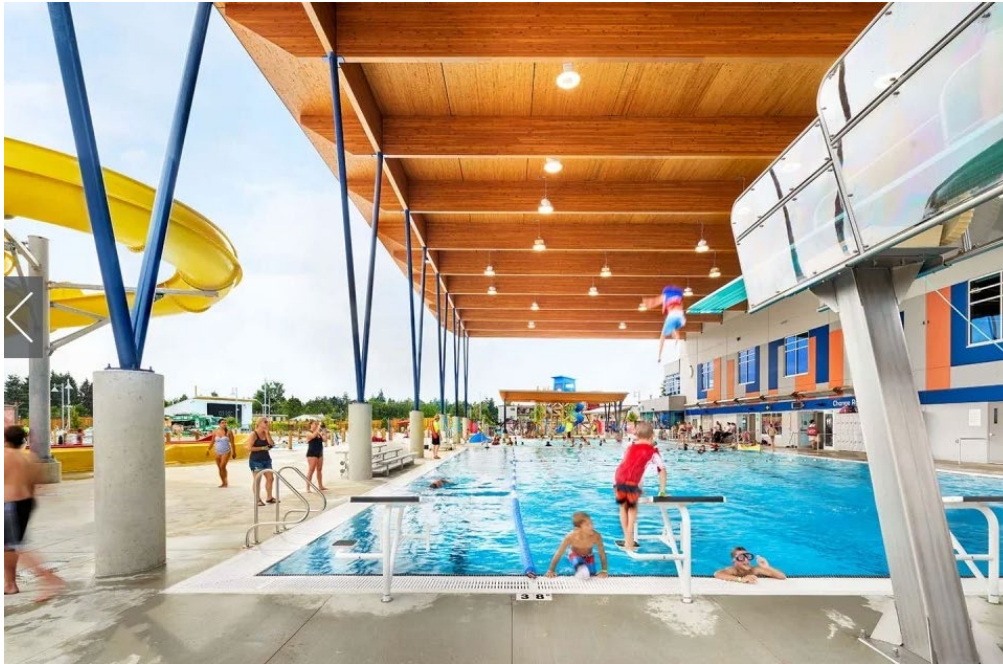
Figure 4: Custom Cantilevered Pool Cover
