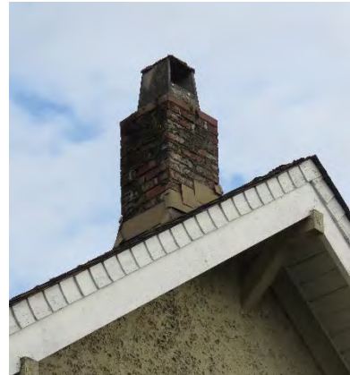
Chimney on west side of the house.
