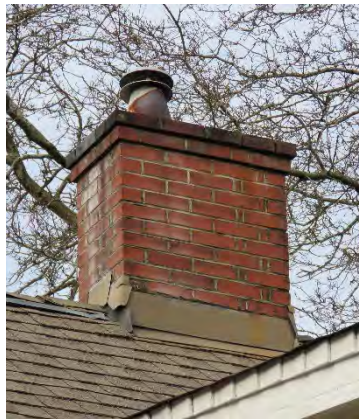
Chimney on east side of the house.
