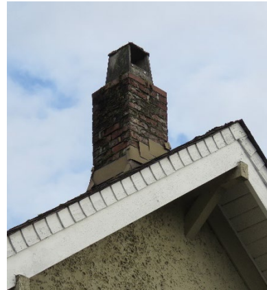
Chimney on west side of the house.
