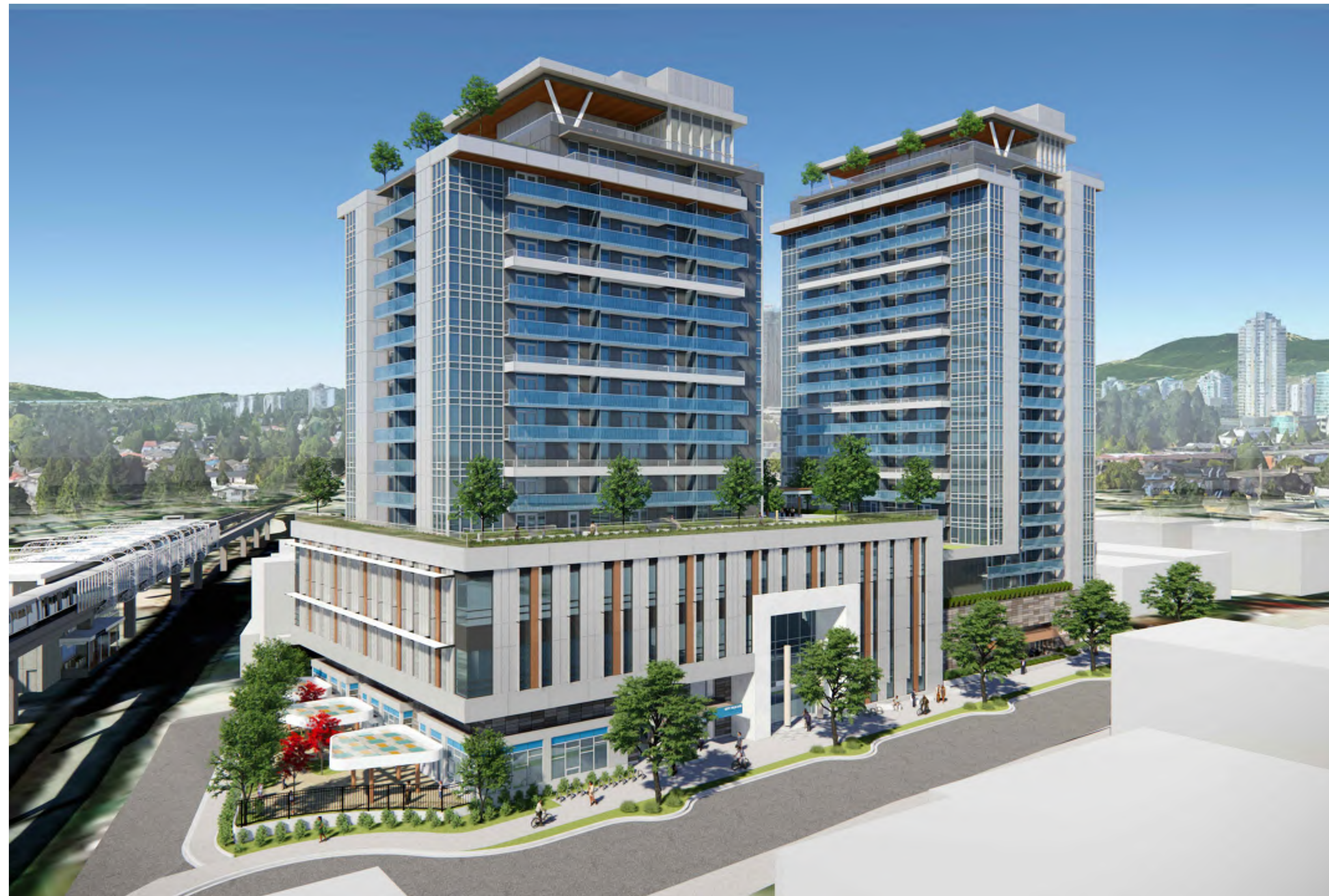
1 SOUTH-EAST ELEVATION VIEW
