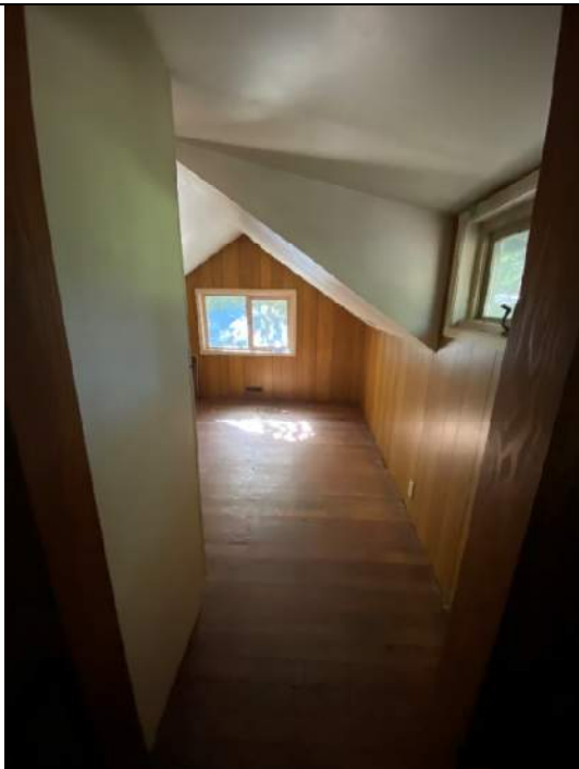
Figure 21: Room in Attic, low ceiling.
