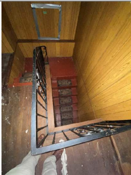
Figure 22: Stairs to Attic, non-original railings.
