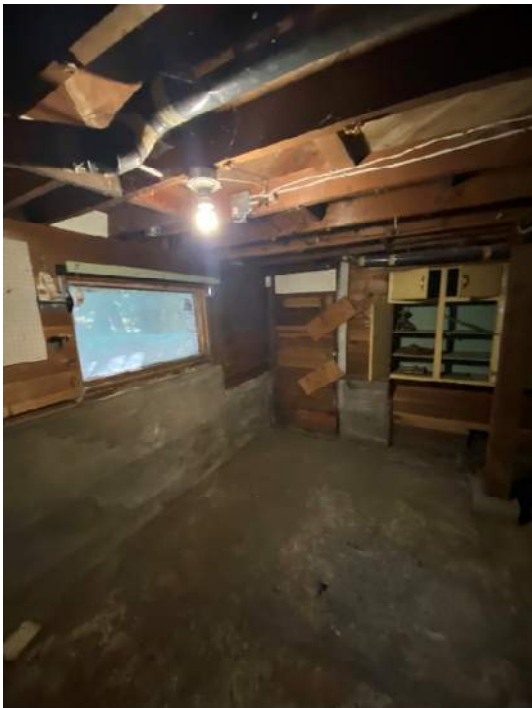
Figure 23: Basement and foundations.
