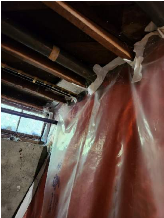
Figure 24: Basement with modern interventions.
