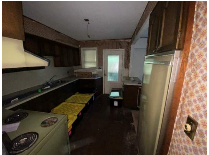
Figure 18: Kitchen, with non-original millwork.
