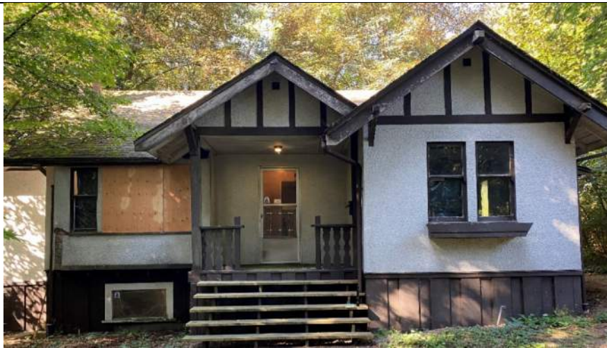
Figure 1: 2023 front entrance to Hill Cottage.
