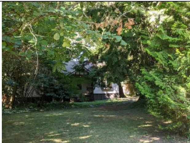
Figure 4: 2023 Street view, east elevation (front of Hill Cottage).
