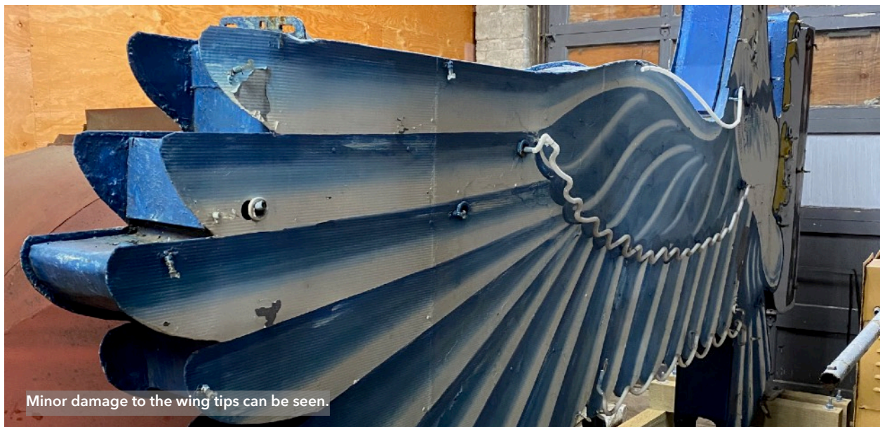
Construction details and the distinctive corrugated sheet metal
