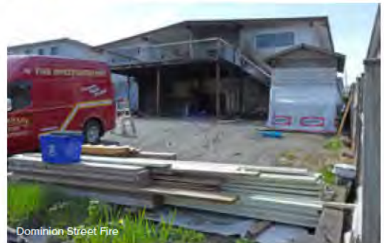
Dominion Street Fire
