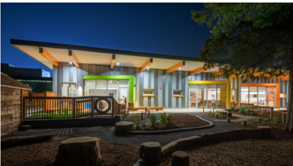
Well-lit secure entry
