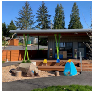
Modular facility at elementary school
