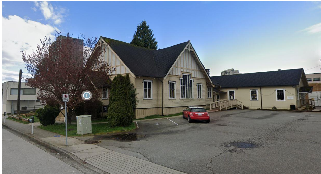
Historic 1912 church at 7135 Walker Avenue in Edmonds, showing a later addition at rear
