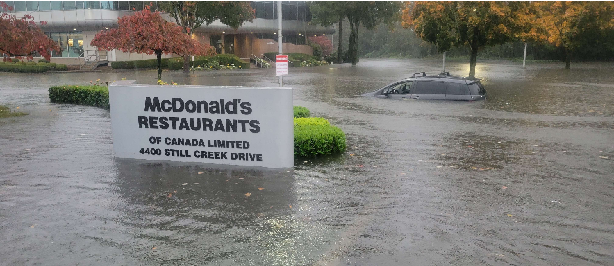
View downstream of Still Creek Drive bridge, Burnaby
