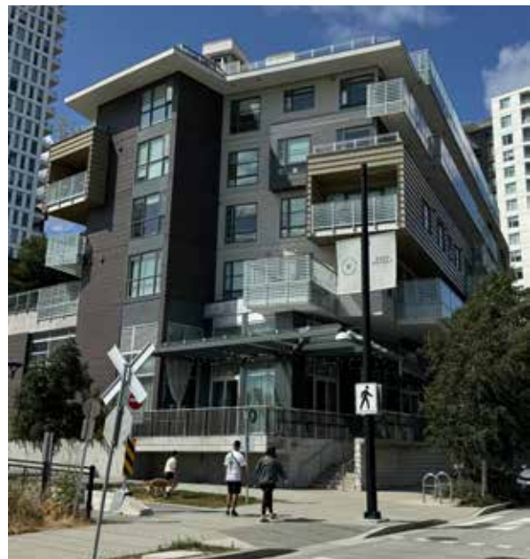
Low-rise mixed-use building in River District, Vancouver
