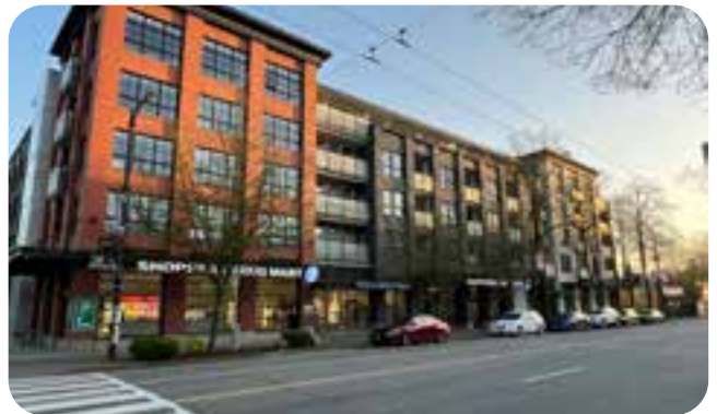
Mixed-use buildings with commercial units at ground level and apartments above
