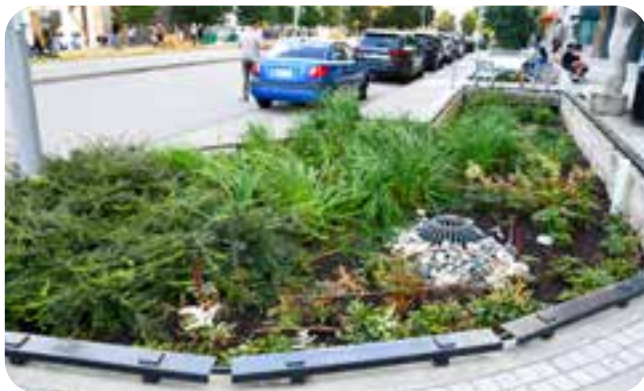
Rain gardens are a type of green infrastructure
