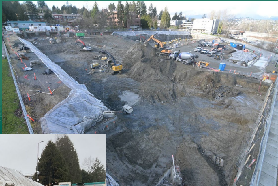
Excavation of Underground Parkade
