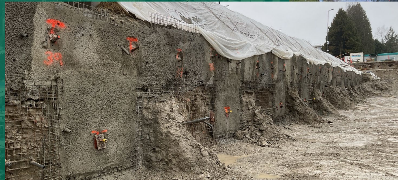
Excavation and Shoring along the Western Property Line
