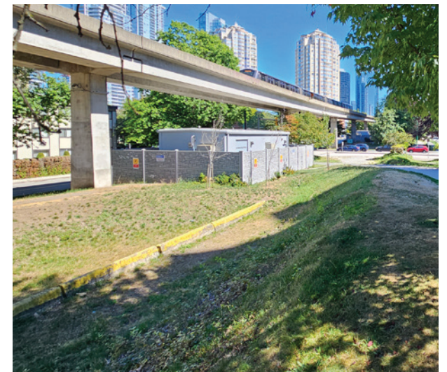
Depressed area and utility structure just east of Willingdon Avenue.
