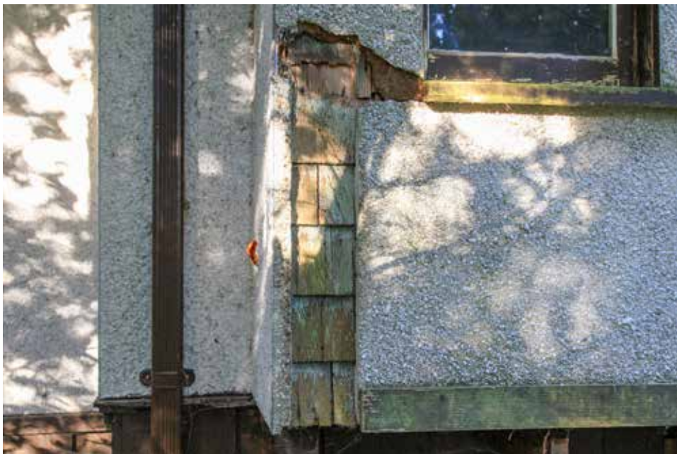
Detail of exposed original wood shingle cladding on the square oriel window on the front elevation of the Hill Cottage.
