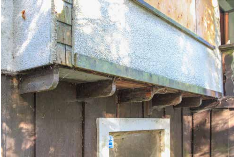
Detail of round corner wood joists below the square oriel window on the front elevation of the Hill Cottage.
