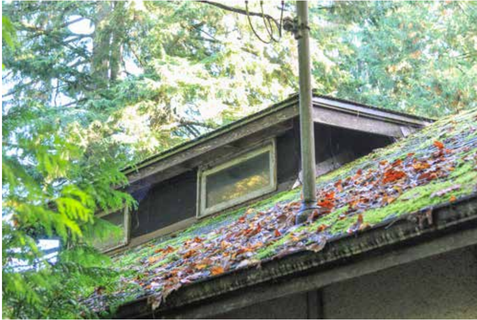
Detail of a low-profile shed-roof dormer on the rear elevation of the Hill Cottage.
