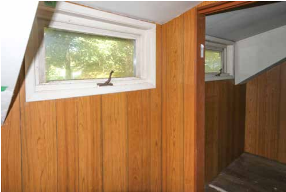
Detail of the two single-light, wood sash windows of the shed-roof dormer from the interior of the Hill Cottage.
