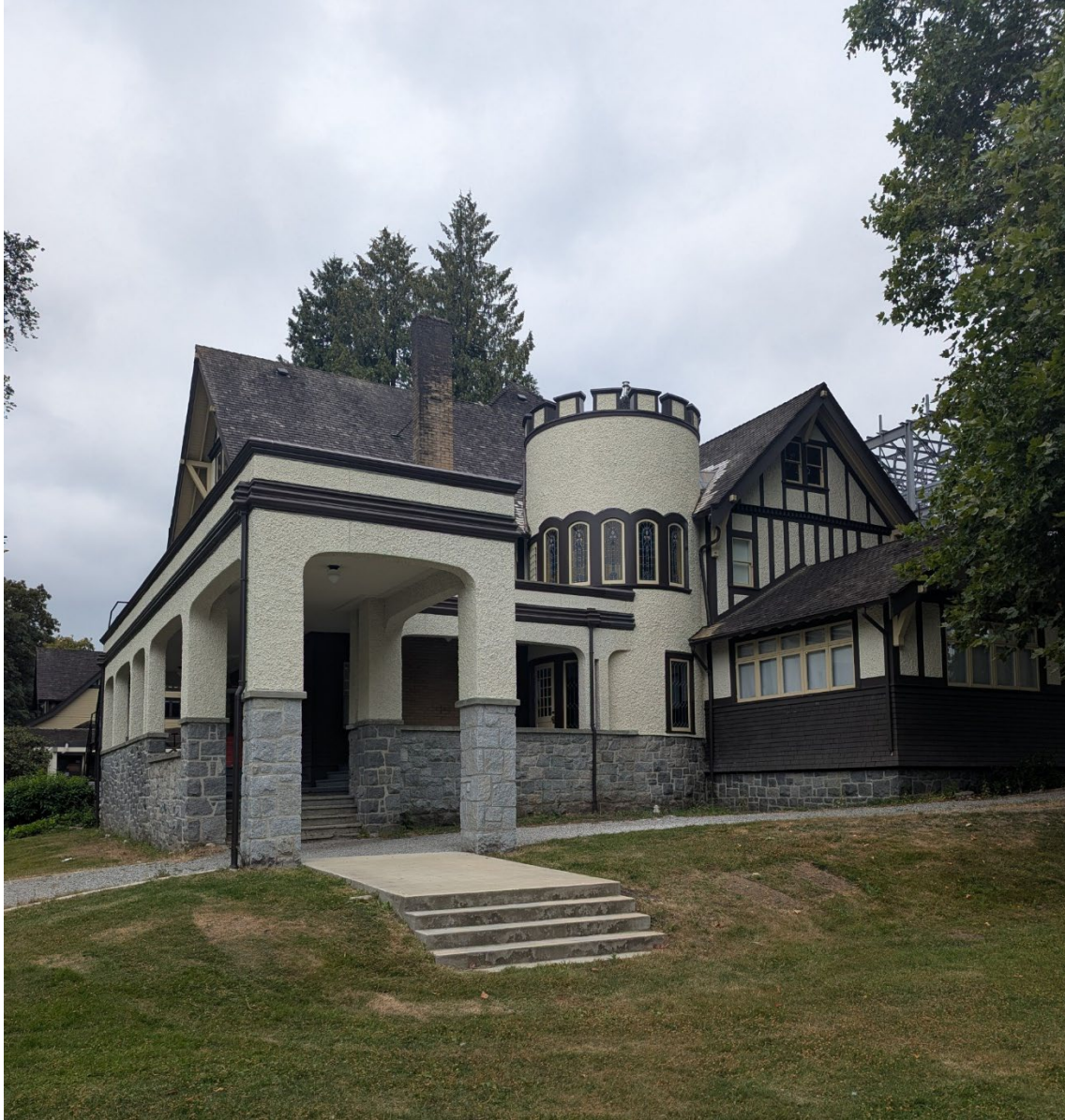
The W.J. Mather Residence after the repair and restoration of the turret and verandah, repointing of the granite foundation walls, and reconstruction of the porte cochere (completed in September 2024).
