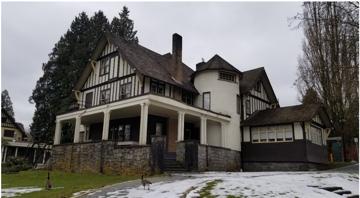
The W.J. Mather house in 2019, prior to restoration of the verandah and turret, and recreation of the original porte cochere.
