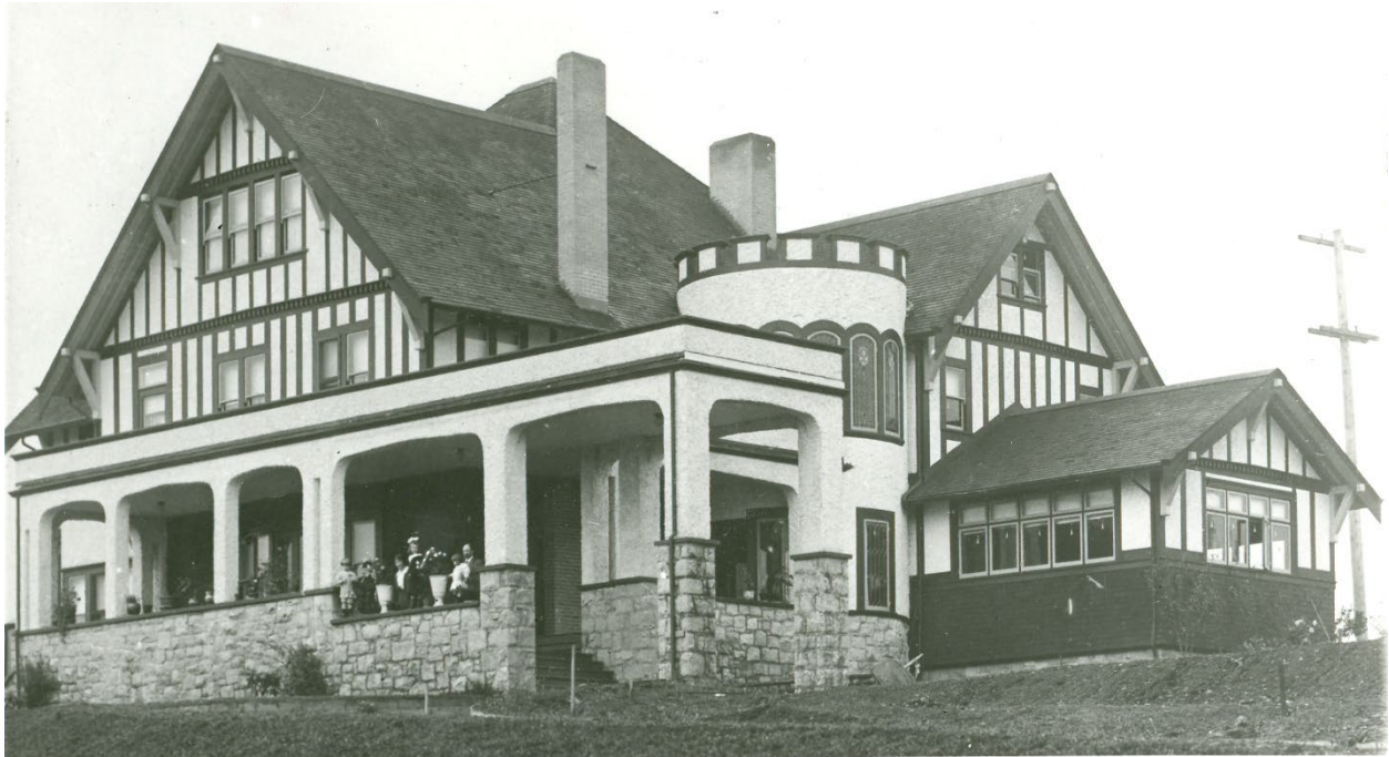
The W.J. Mathers house in 1912. The original cedar shingle roof and two of three original chimneys are visible in the photograph. PHOTO: HV985.57.1 (BURNABY VILLAGE MUSEUM).
