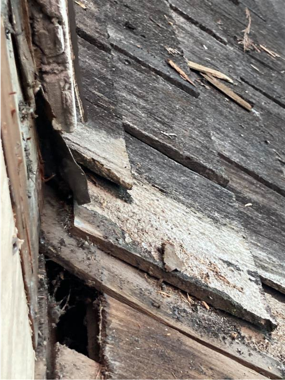
Detail of the shingles, prior to replacement.
