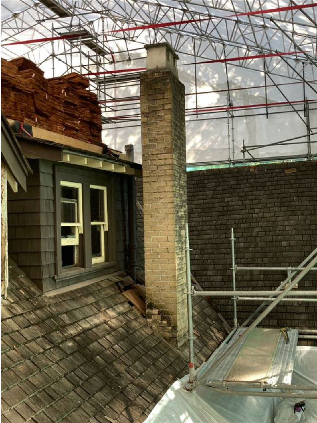
A photograph from early 2024 shows the condition of the roof prior to replacement of the shingles. Replacing the flashing between the chimney and the roof was part of the scope of the project.
